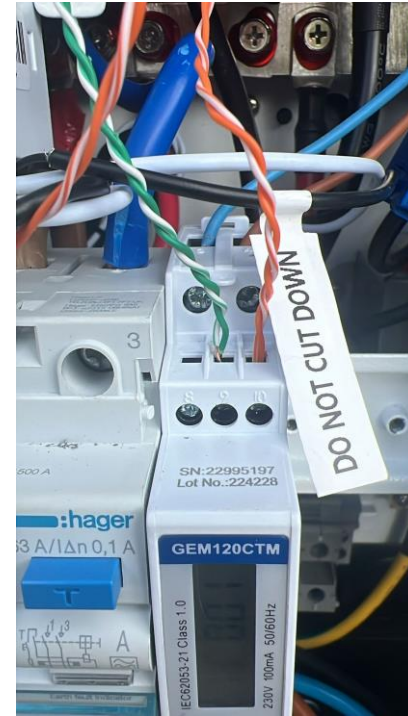
Here 1 pair used for A and 1 for B - INCORRECT
