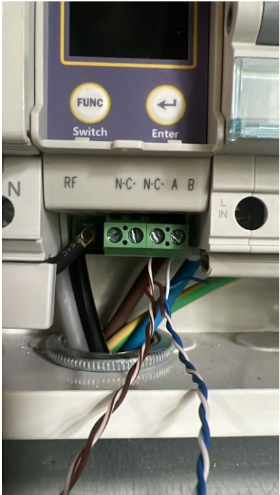
Here is 1 wire from 2 pairs - INCORRECT
