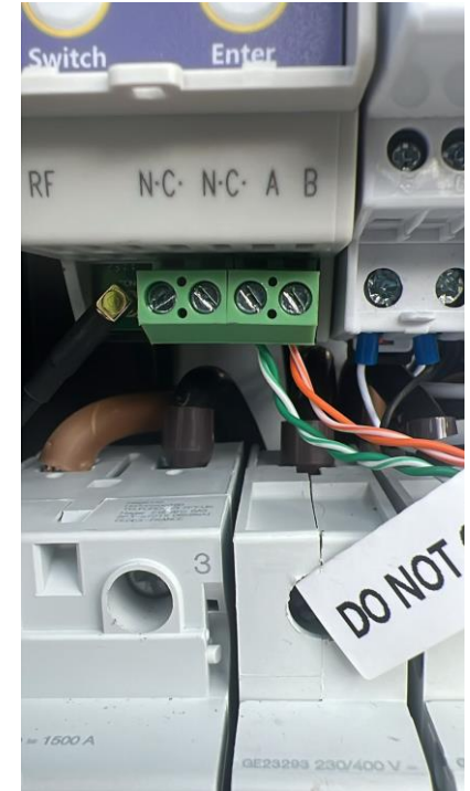
Here 1 pair used for A and 1 for B - INCORRECT
